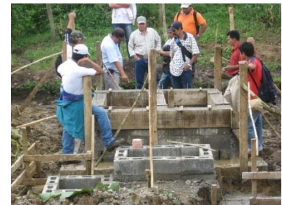
Construction of CPFs during the project
